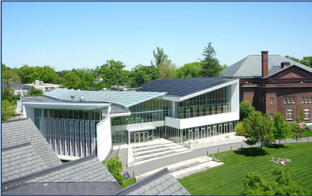
Community Energy's Smith College Solar Project- Northampton, MA
